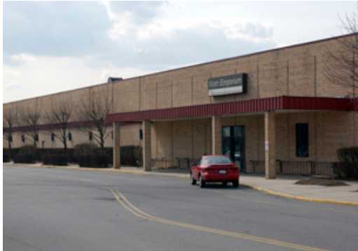
Figure 1. Street View of the Math Emporium
